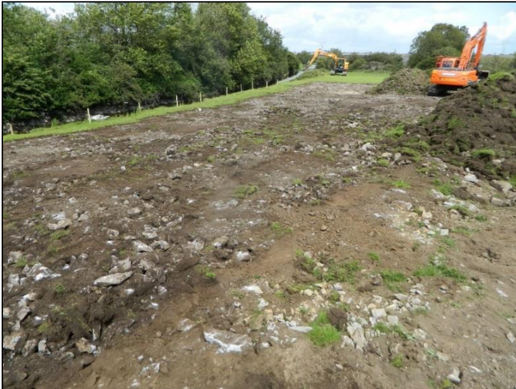
Plate 1 Facing northeast showing topsoil strip along riverbank southeast of Dunkellin Bridge
