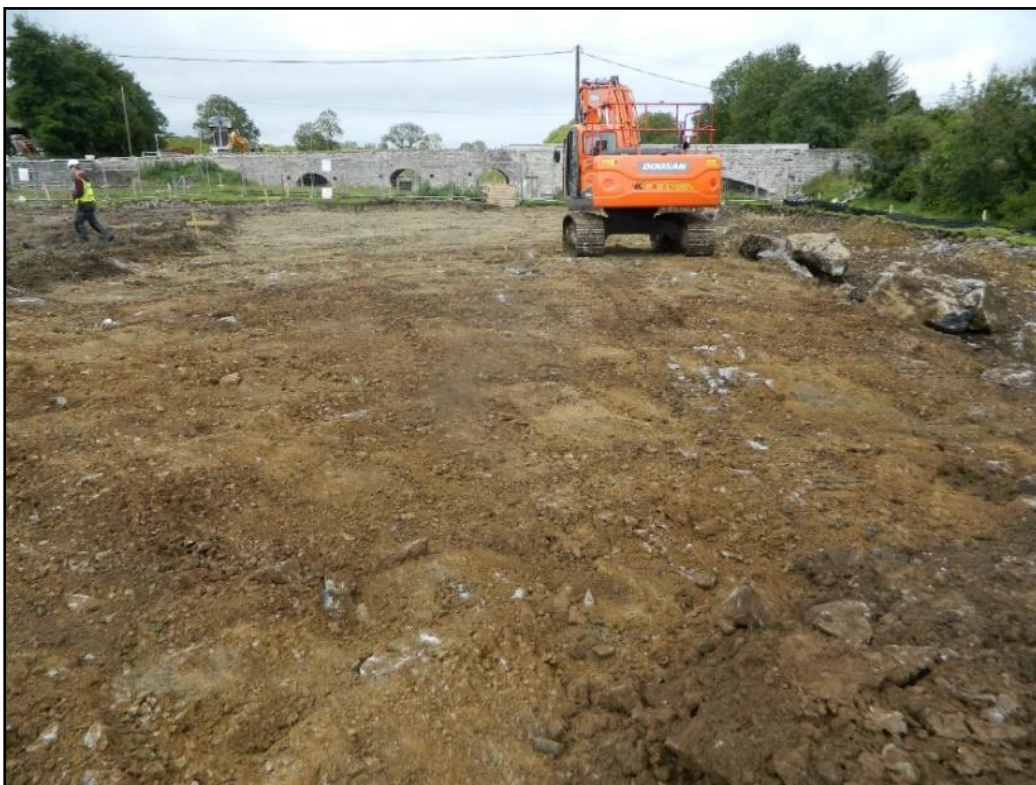
Plate 2 Facing west towards Dunkellin Bridge showing exposed rocky ground in foreground and soft silty clay in background
